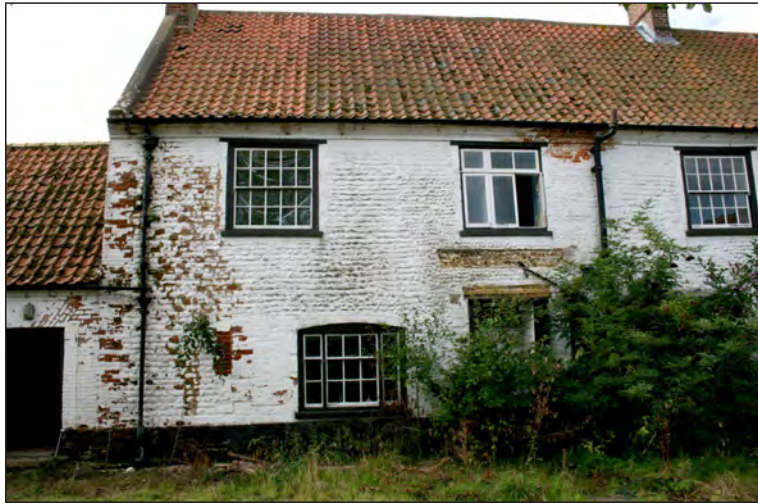
Plate 5. Relocated ground floor window on northern elevation of Building A
