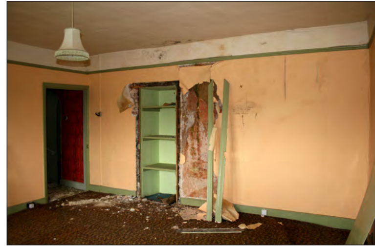
Plate 26. Niche indicating previous doorway in Building A
