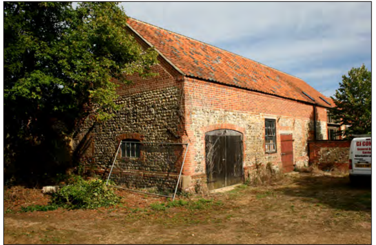
Plate 44. Building G facing north-west
