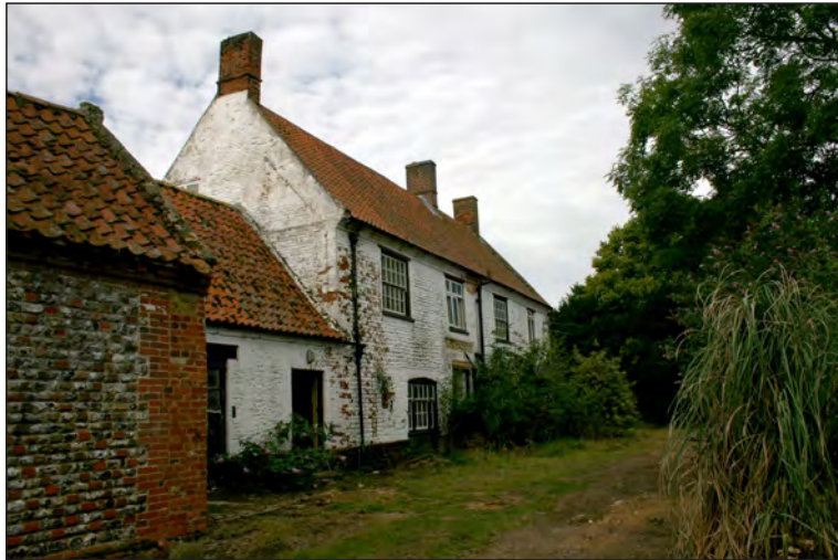
Plate 1. Building A, north elevation facing south-west
