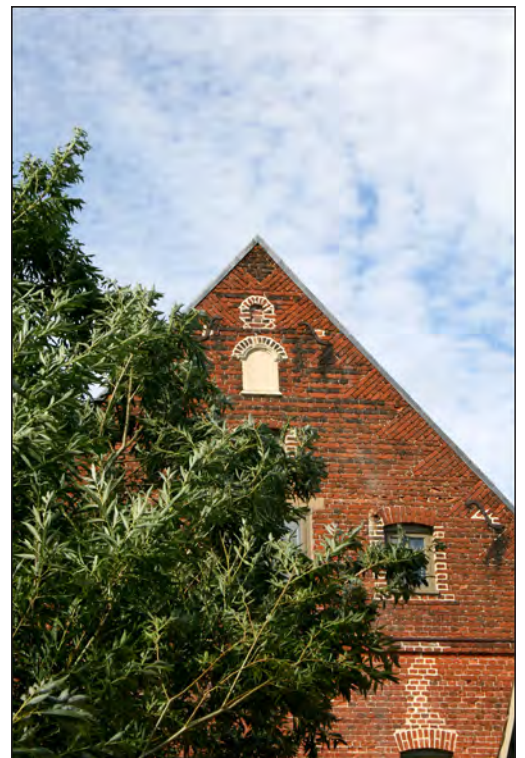
Plate 52. Ivy Farm barn southern elevation
