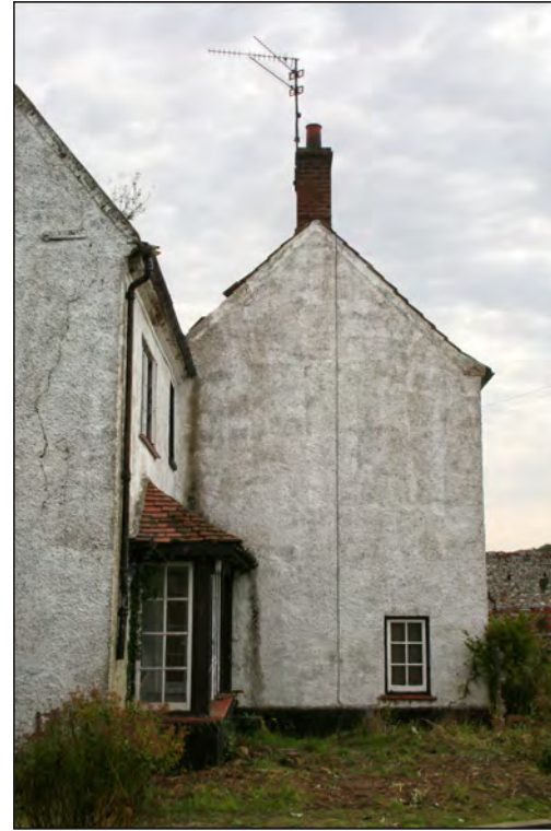
Plate 14. Western elevation of Building B
