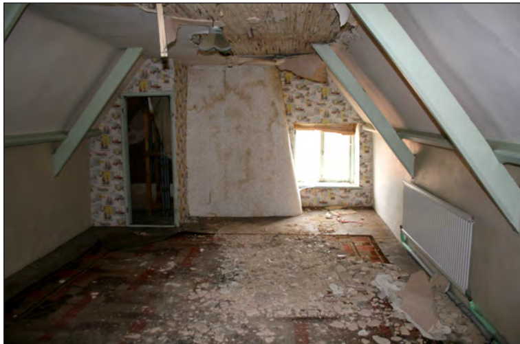
Plate 27. Second floor east bedroom
