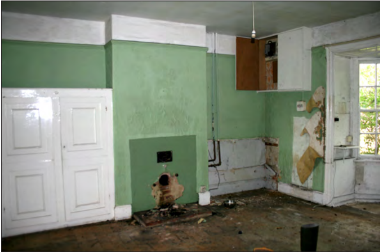
Plate 21. Central ground floor room, Building A
