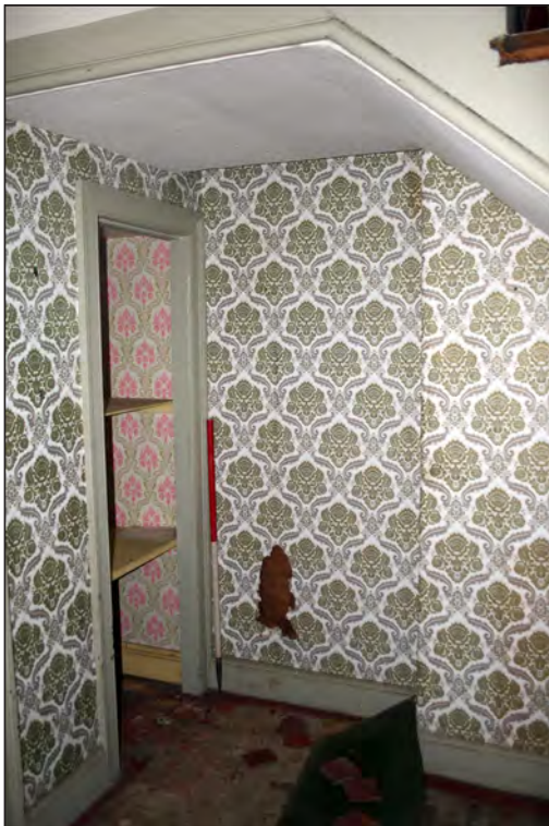
Plate 19. Blocked doorway beneath stairs in Building A, 1m scale
