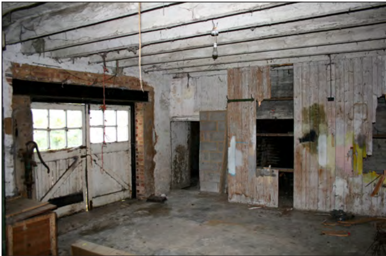
Plate 35. Interior of Building C, fireplace to right
