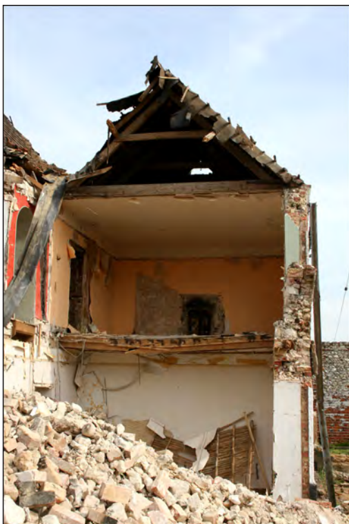
Plate 29. Construction of Building B's walls
