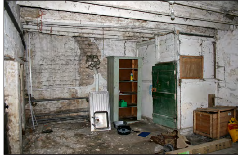
Plate 34. Interior of Building C, west end
