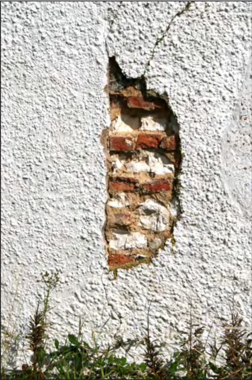
Plate 9. Exposed walling on west elevation of Building A
