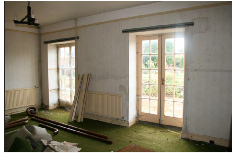
Plate 18. French windows, ground floor, Building B
