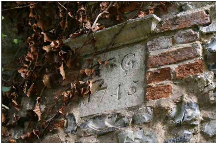
Plate 47. Date stone above blocked door on Building G
