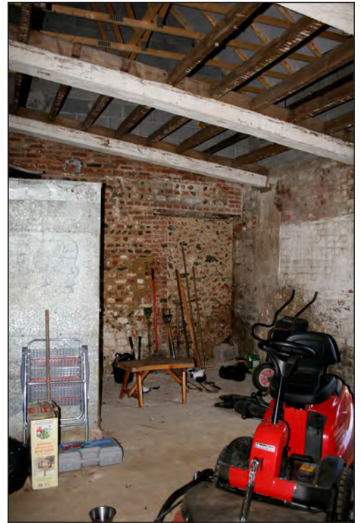
Plate 50. Blocked door in northern wall of northern cell, Building G
