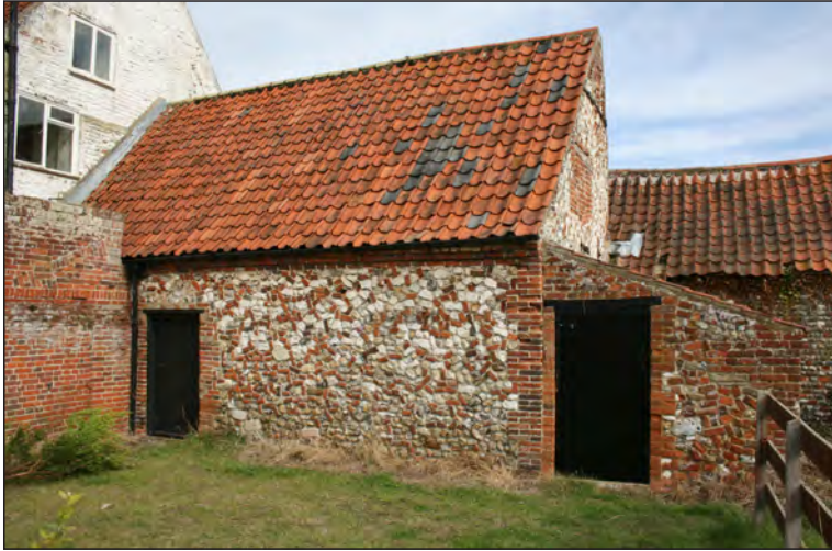
Plate 33. Southern elevation of Building C
