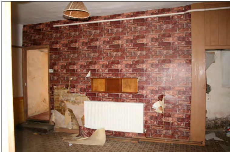
Plate 15. Boarded up fire-place in eastern ground floor room, Building A
