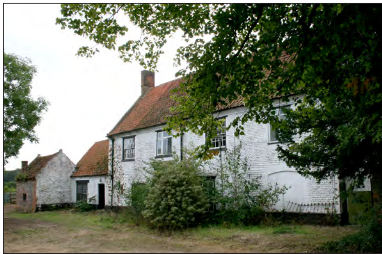
Plate 3. Building A north elevation facing south-east
