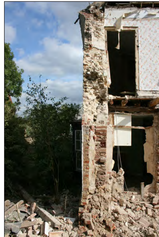
Plate 28. Construction of Building A's walls
