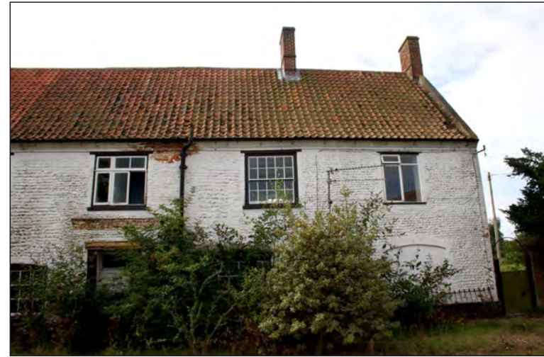
Plate 6. In-filled window on northern elevation of Building A
