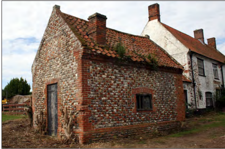
Plate 37. Building D facing south-west
