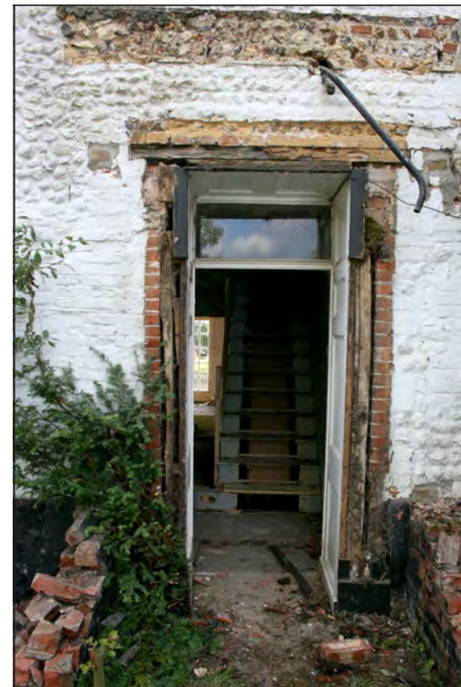
Plate 4. Front door with porch surround removed
