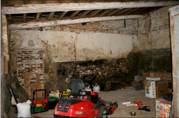
Plate 49. Interior of northern cell Building G
