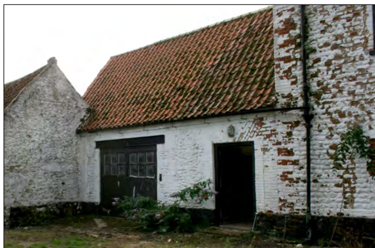
Plate 31. Building C north elevation
