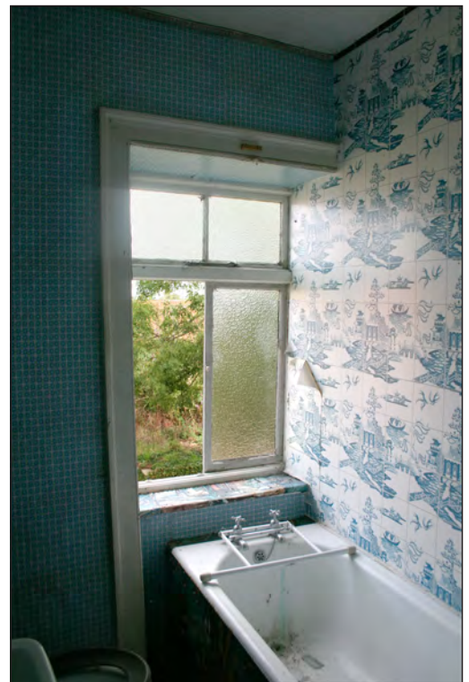
Plate 24. Window divided by partition wall in Building A
