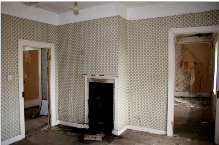
Plate 23. Fire-place first floor central bedroom Building A
