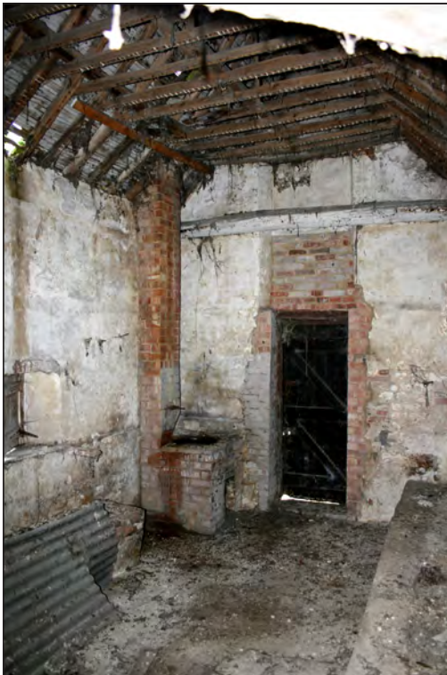
Plate 39. Interior of Building D
