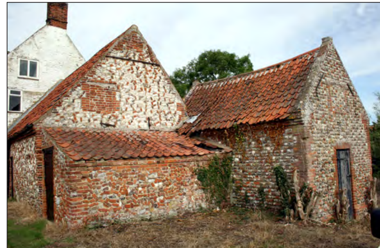
Plate 40. Building E east elevation
